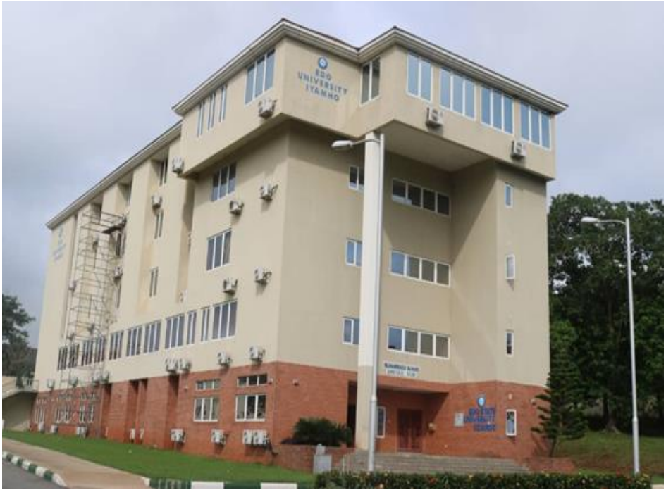
University Administrative Building
